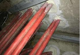
Figure 7. Silicone and foam used to stop water ingress
