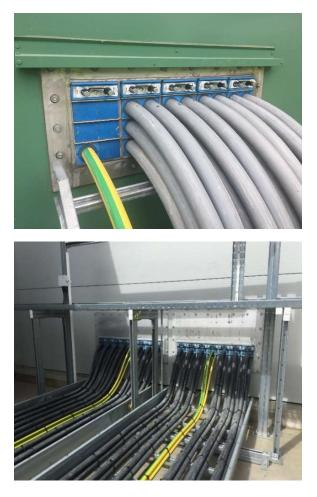
Figure 10. Large area building penetrations for power systems sealed against water ingress
