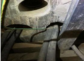
Figure 6. Unsealed ducts quickly fill with water and debris
